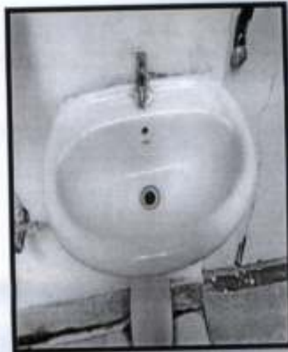
Water efficient Taps
